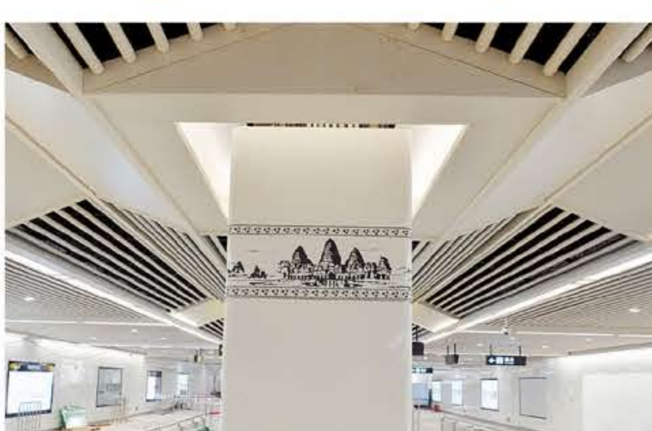
Application of UHPC in underground decorative panels
