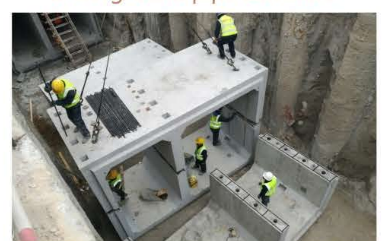
Application of UHPC in underground pipe corridors
