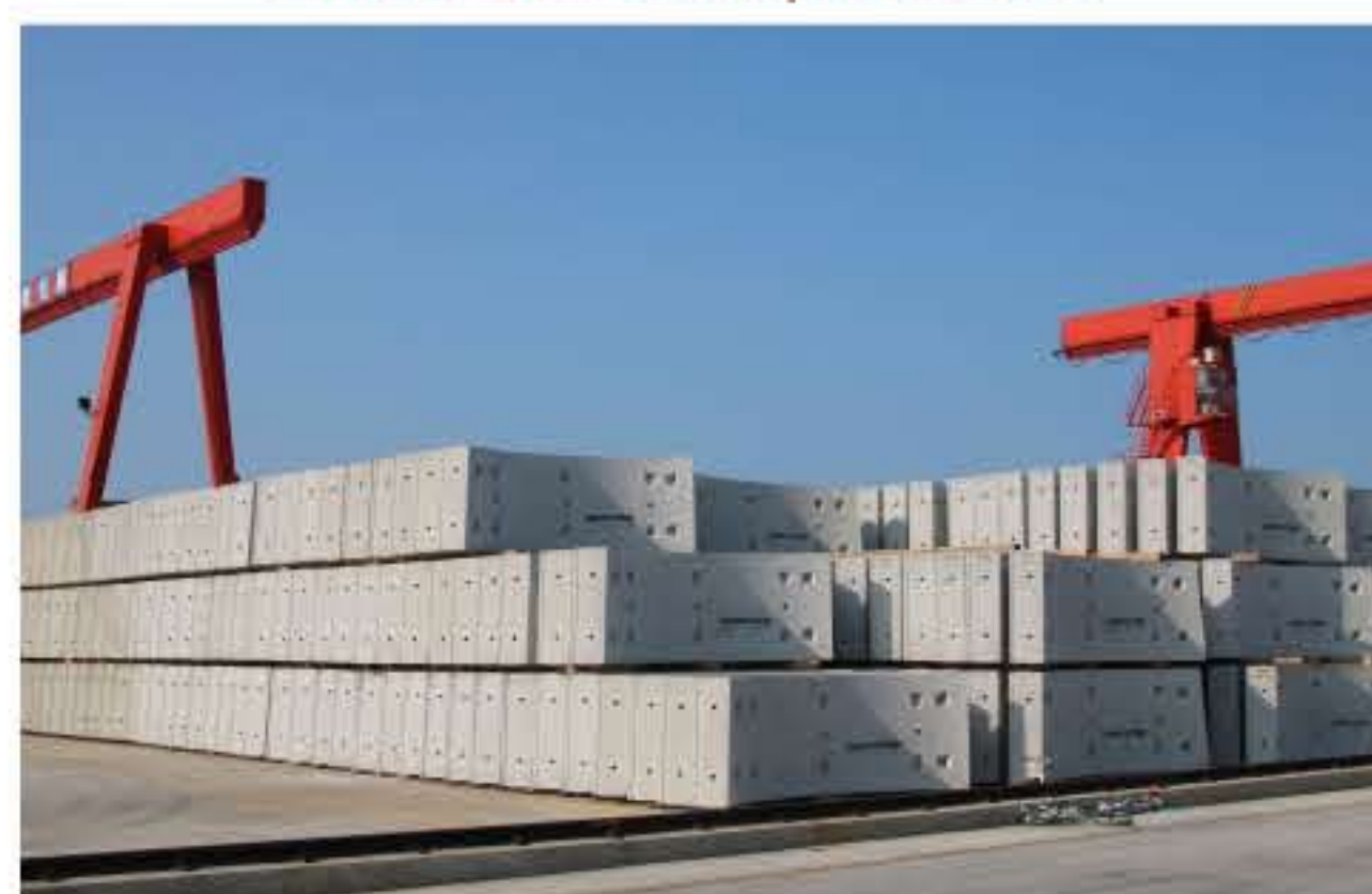
Application of UHPC in precast concrete components
