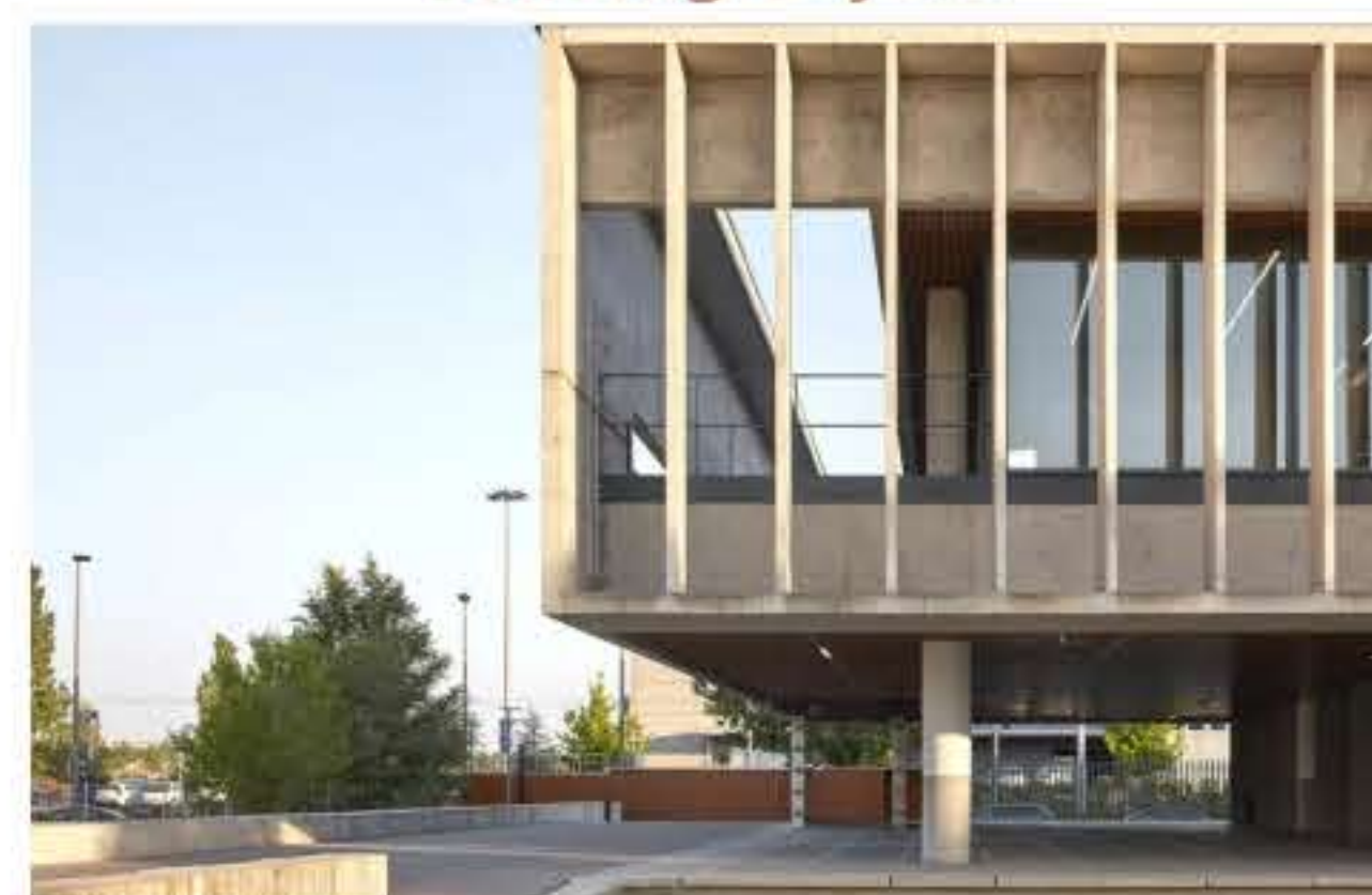
UHPC in Seismic Columns for Building Foyers
