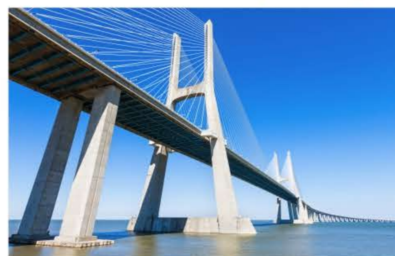
Application of UHPC in anchor zone concrete of cable-stayed bridges
