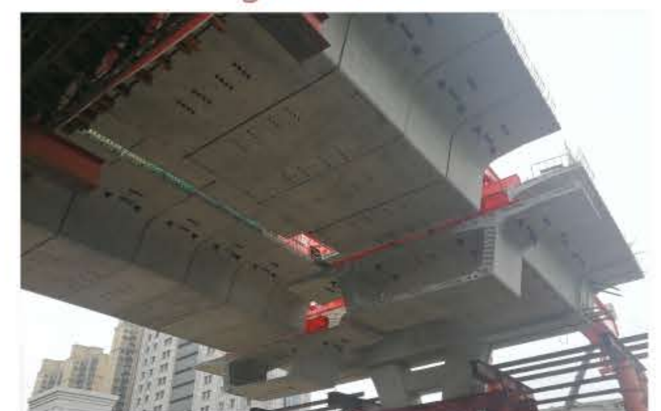
Application of UHPC in precast girder box
