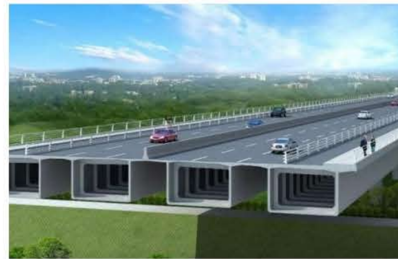
UHPC in thin-walled cover beams
