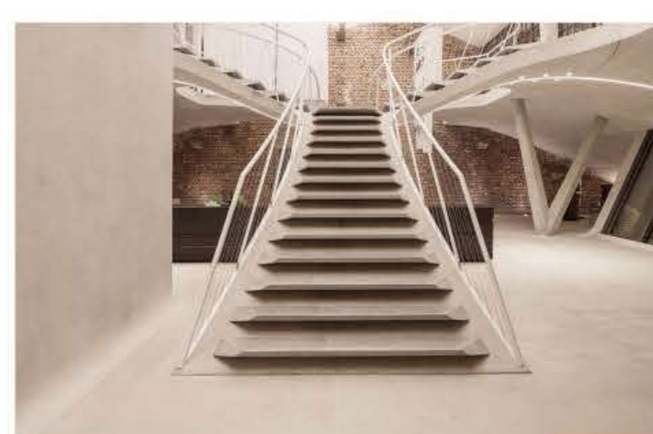
UHPC in lightweight staircases
